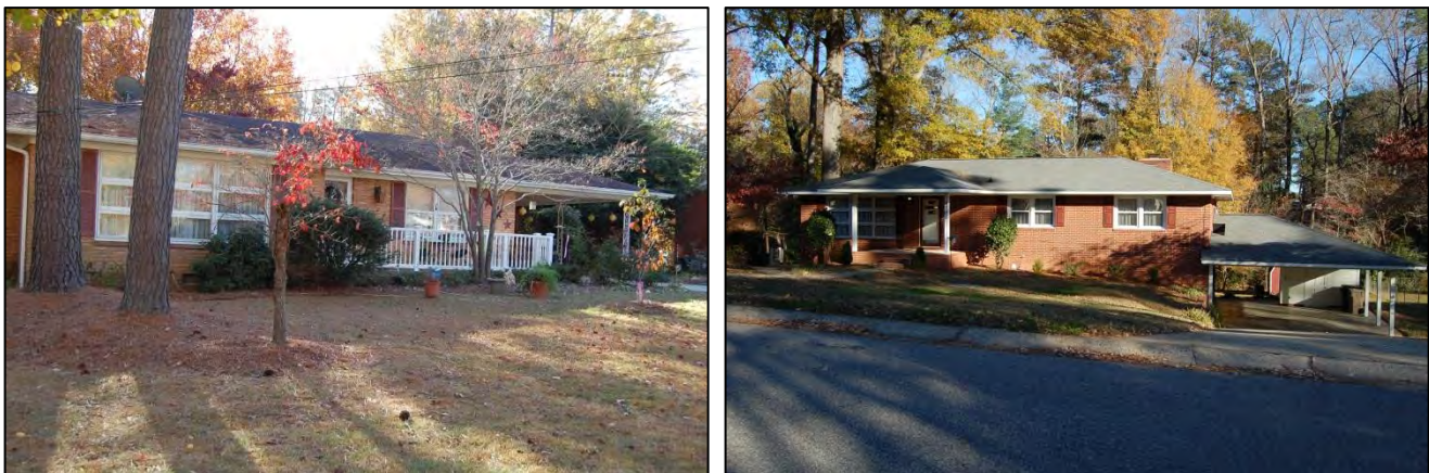
Figure 14. Ranch houses with nine-horizontal-light picture windows at 405 Roxanne, at left, and 4705 Forestdale, at right
