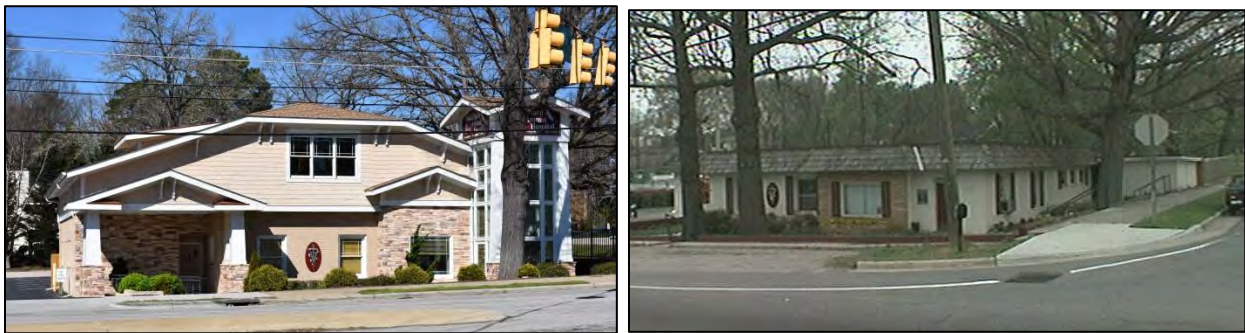
Figure 90. Boulevard Animal Hospital at 3900 Western Boulevard, Raleigh (1948, 2012): current image, at left, and 1996 tax record image, at right (source: http://www.wakegov.com/gis/imaps )
