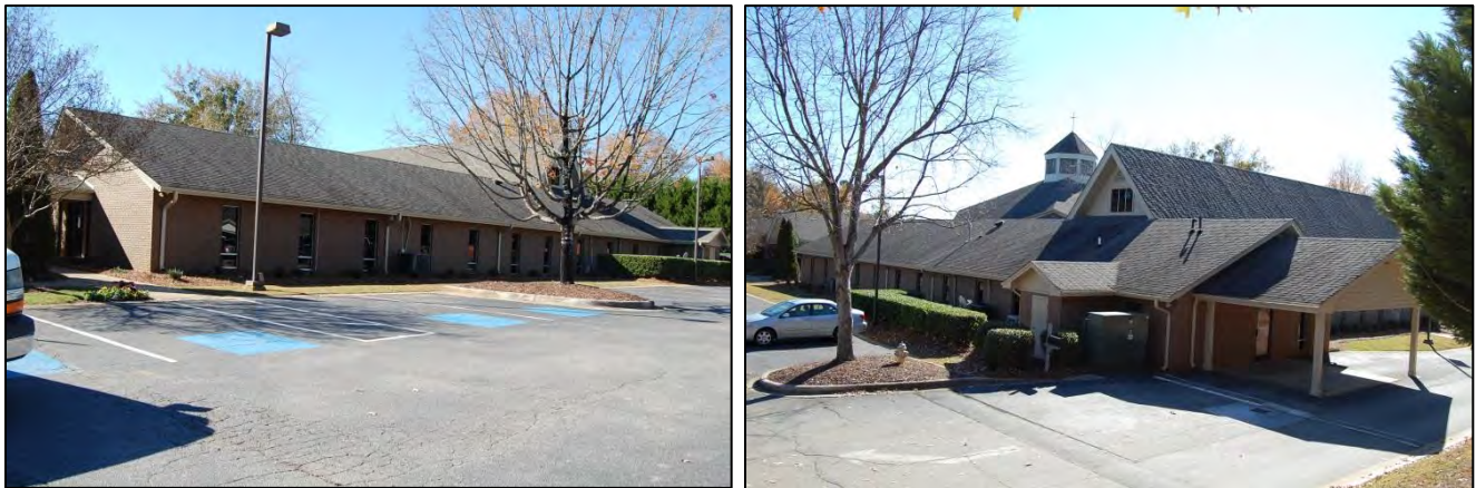
Figure 71. Original Capital Pentecostal Holiness Church, east side and north rear elevations, at left, and north rear and west side elevations, at right; note modern windows and porte cochere and attached newer sanctuary
