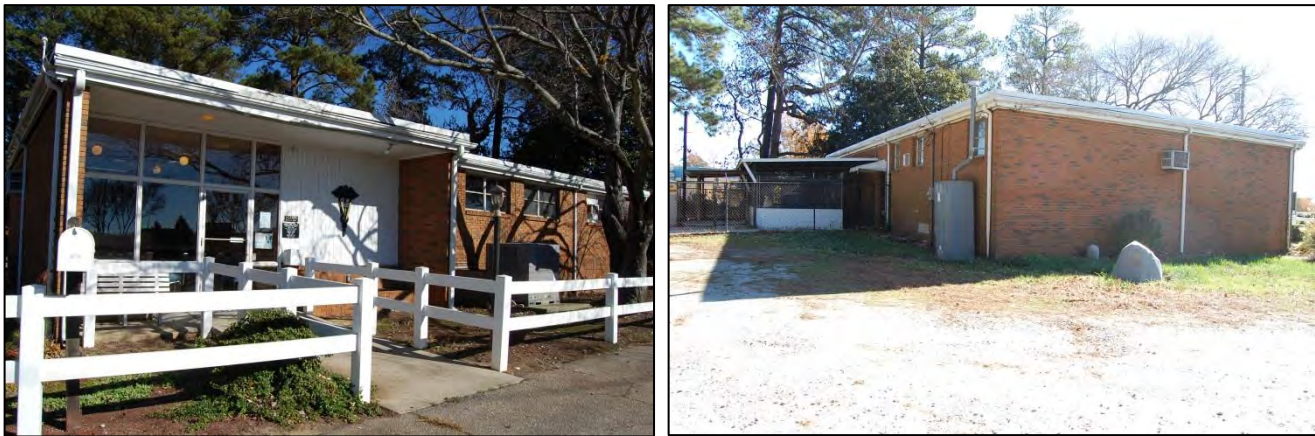
Figure 85. Garner Animal Hospital: south front and west side elevations, at left, and west side and north rear elevations, at right
