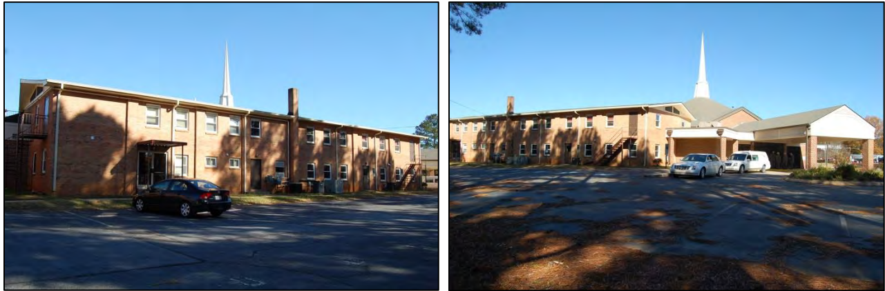
Figure 62. West gable and south rear elevation of original education/social block, at left, and east gable and south elevation, at right
