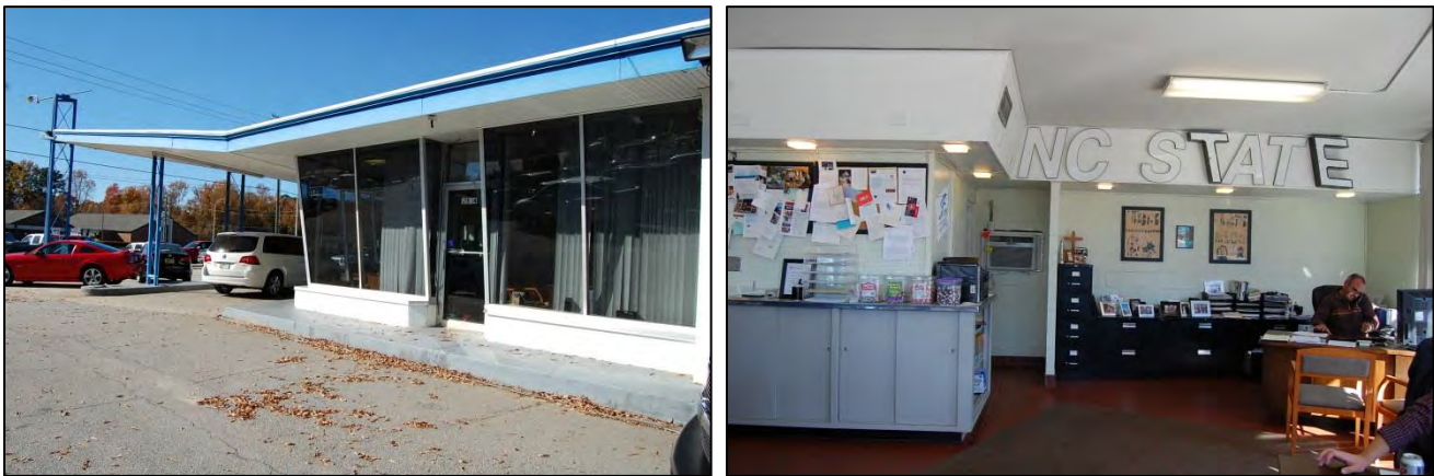
Figure 52. Looking southwest at east side elevation of office, at left, and at office interior, at right
