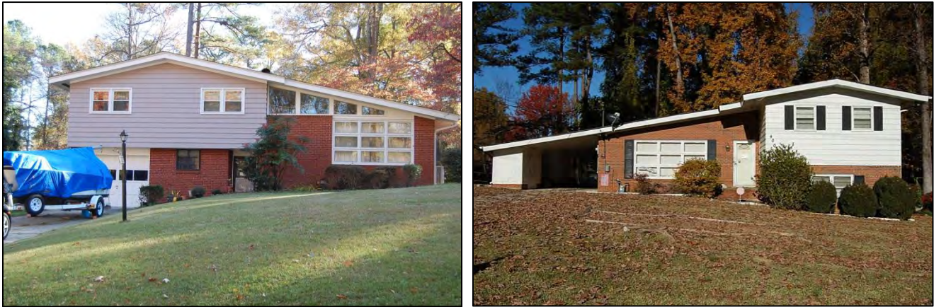
Figure 28. Mid-century-modern-influenced split-level houses at 619 Winterlochen, at left, and 400 Winterlochen, at right
