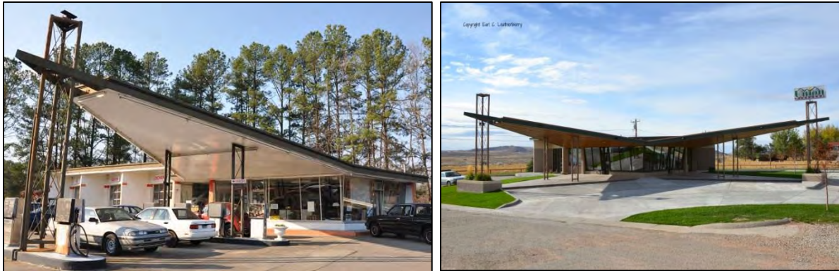
Figure 55. Extant former three-service-bay station in Sanford, NC, no date, at left (source: http://www.roadarch.com/10/3/p66.jpg ; renovated double-canopy, two-service-bay station in Rawling, WY in 2015 (source: https://www.flickr.com/photos/23711298@N07/23854693124/in/pool-1396109@N22/ , photographer: Earl Leatherberry)
