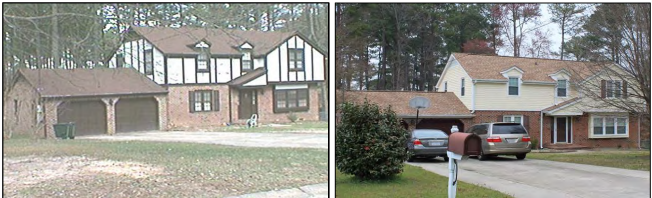
Figure 30. Non-contributing split-level at 5004 Cindy, appearance in 1996, at left, and now, at right; note replacement of faux Tudor Revival-style half-timbering and stucco with synthetic siding (source of 1996 photograph: http://www.wakegov.com/gis/imaps )
