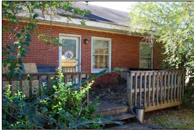
Figure 73. Former Capital Pentecostal Holiness Church parsonage: north rear elevation
