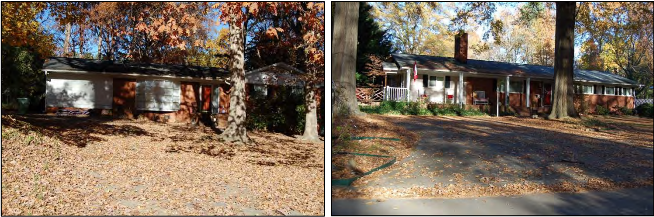
Figure 24. 4408 Susan, at left, with carport converted into room, and 510 Roxanne, at right, with converted carport and altered picture window and porch posts; both recommended as non-contributing
