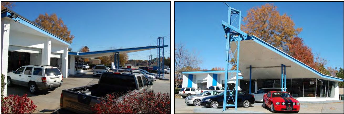
Figure 50. Looking east at front elevation, at left, and to north, at right
