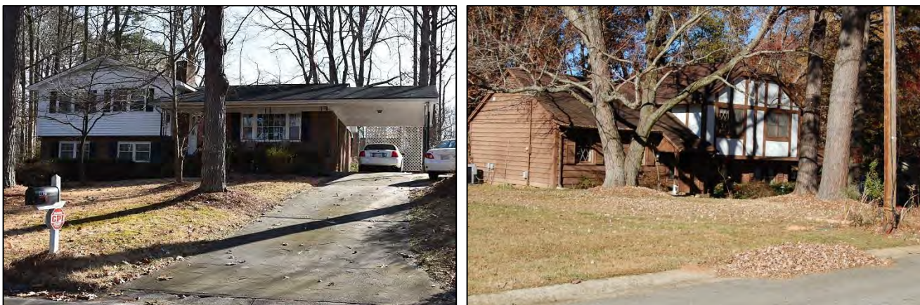
Figure 27. 4921 Cindy, at left, with original bay window and carport, and 4812 Comelia, retaining original Tudor Revival-style windows and faux half-timbering and stucco
