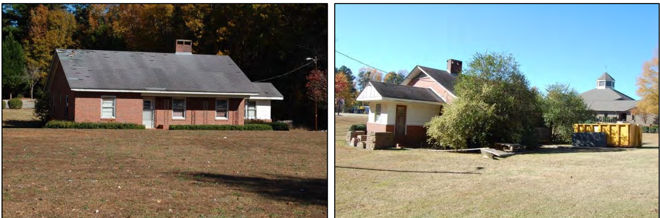
Figure 72. Former Capital Pentecostal Holiness Church parsonage: west side and south front elevations at left, and east side and north rear elevations, at right
