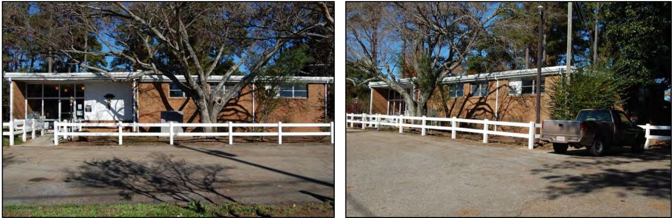
Figure 84. Garner Animal Hospital: south front elevation, at left, and south front and east side elevations, at right
