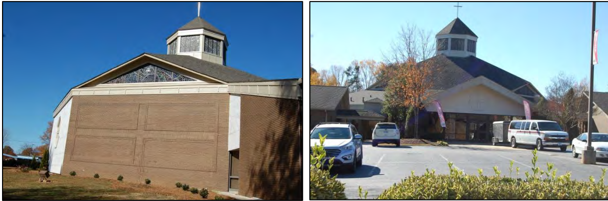
Figure 75. Second sanctuary: southeast elevation, at left, and north elevation, at right
