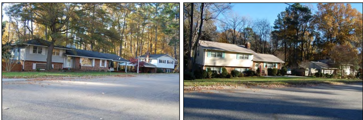
Figure 9. Split-level houses at 4716 and 4712 Greenbrier (L to R), at left, and 4713 and 4717 Forestdale (L to R), at right
