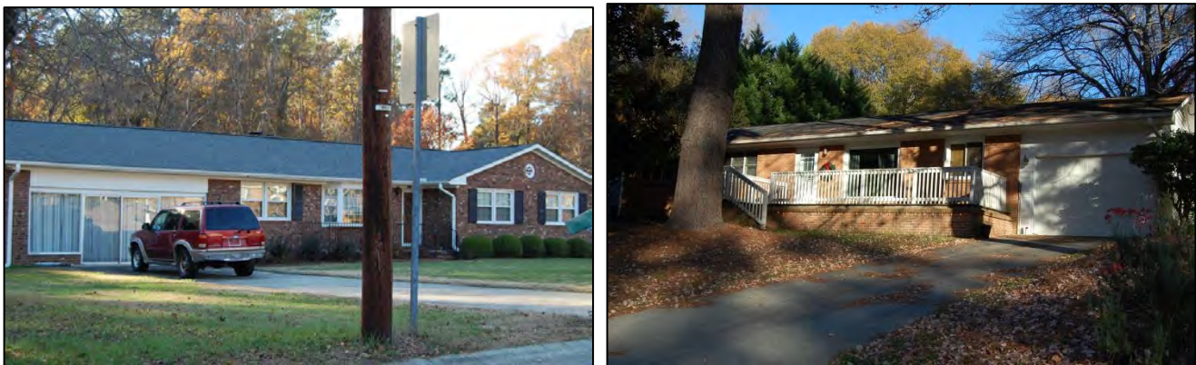
Figure 23. 4810 Greenbrier, at left, with carport converted into glass-fronted room, and 4409 Greenbrier, at right, with carport converted into garage and bay window altered; both recommended as non-contributing
